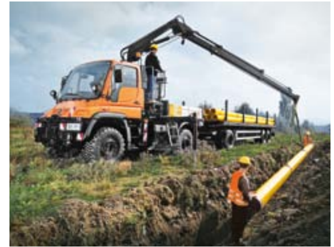
Its versatility makes the Unimog an all-round expert in pipeline construction.
