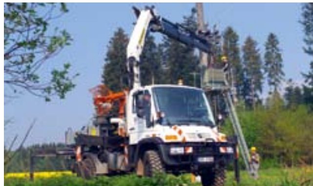
Maintenance of overhead lines in rough terrain.
