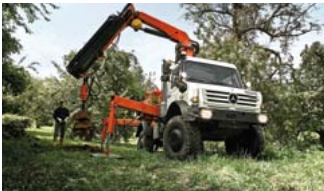
Unimog with digger derrick for mast erecting.
