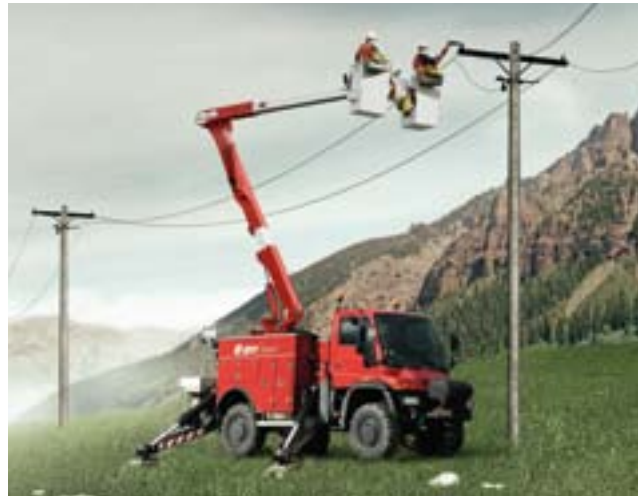
Relaxed working under high tension – on an insulated work platform.
