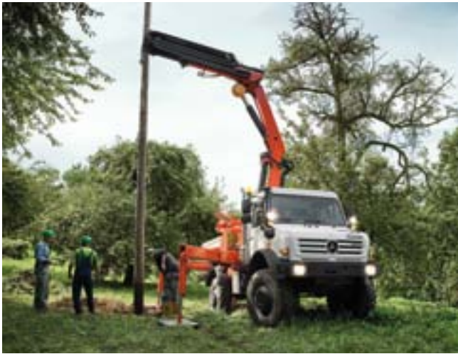
Powerful cranes make erecting steel towers simple.
